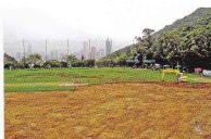
The beginning of the project, excavation of the soil based ground
