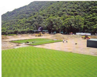
Start of the sub-base levelling
