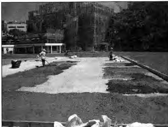
Laying of black clay.
